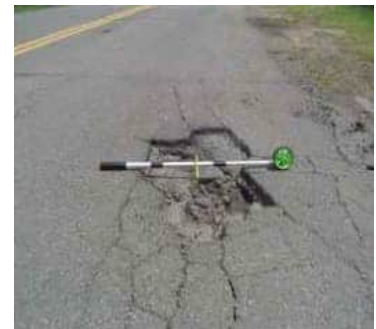
Figure 32 High Pothole PAVER™ Distress Identification Manual
