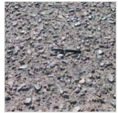
Figure 5 High Weathering PAVER™ Distress Identification Manual
