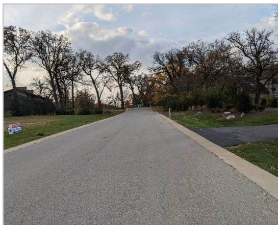
Figure 4 Good Roadway Condition Equestrian Way
