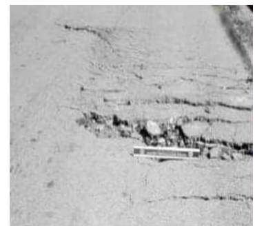
Figure 14 High Slippage PAVER™ Distress Identification Manual
