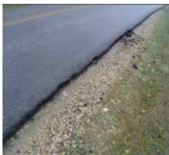
Figure 36 Low Drop-Off PAVERTM Distress Identification Manual
