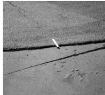
Figure 10 Medium Shoving PAVER™ Distress Identification Manual
