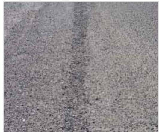
Figure 2 High Raveling PAVER™ Distress Identification Manual
