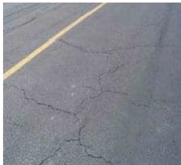
Figure 22 Medium Block Cracking PAVER™ Distress Identification Manual
