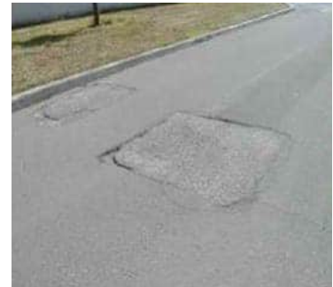
Figure 35 High Patch PAVERTM Distress Identification Manual
