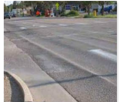
Figure 8 High Rutting PAVER™ Distress Identification Manual
