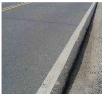
Figure 37 Medium Drop-Off PAVERTM Distress Identification Manual
