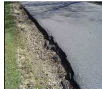
Figure 38 High Drop-Off PAVERTM Distress Identification Manual
