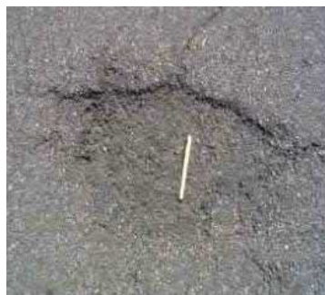
Figure 30 Low Pothole PAVER™ Distress Identification Manual
