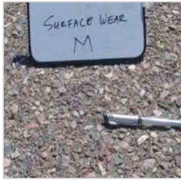
Figure 4 Medium Weathering PAVER™ Distress Identification Manual
