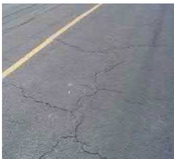
Figure 22 Medium Block Cracking PAVER™ Distress Identification Manual
