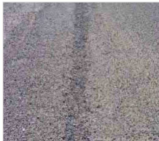
Figure 2 High Raveling PAVER™ Distress Identification Manual
