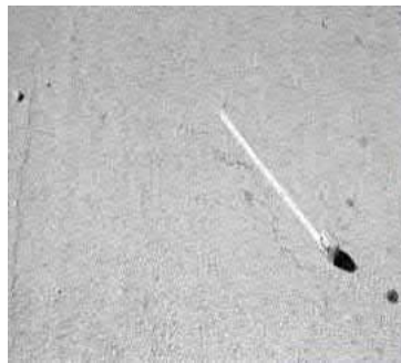
Figure 12 Low Slippage PAVER™ Distress Identification Manual
