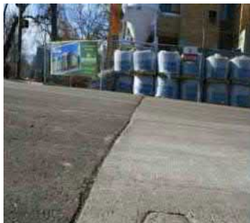
Figure 9 Low Shoving PAVER™ Distress Identification Manual
