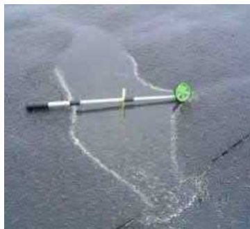
Figure 16 Medium Depression PAVER™ Distress Identification Manual
