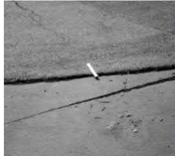
Figure 10 Medium Shoving PAVER™ Distress Identification Manual
