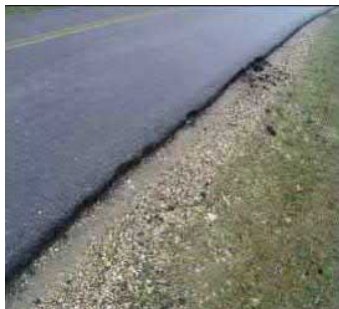
Figure 36 Low Drop-Off PAVERTM Distress Identification Manual
