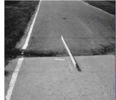
Figure 11 High Shoving PAVER™ Distress Identification Manual
