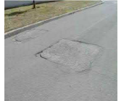
Figure 35 High Patch PAVERTM Distress Identification Manual
