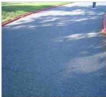
Figure 21 Low Block Cracking PAVER™ Distress Identification Manual
