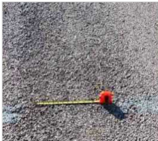
Figure 1 Low to Medium Raveling PAVER™ Distress Identification Manual
