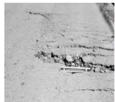
Figure 14 High Slippage PAVER™ Distress Identification Manual
