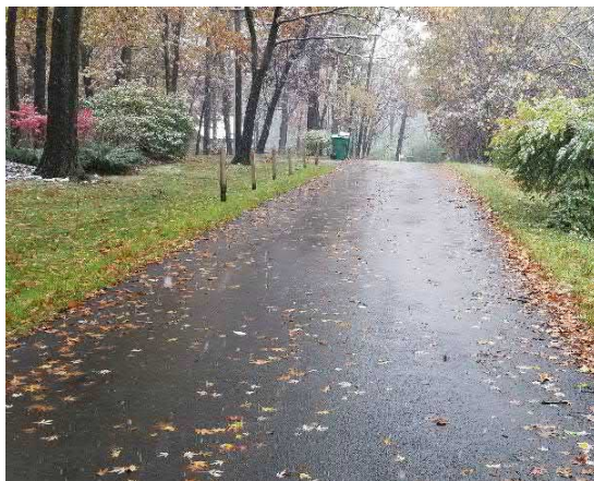
Figure 40 Good Roadway Condition Oak Lane, Lemont, Illinois
